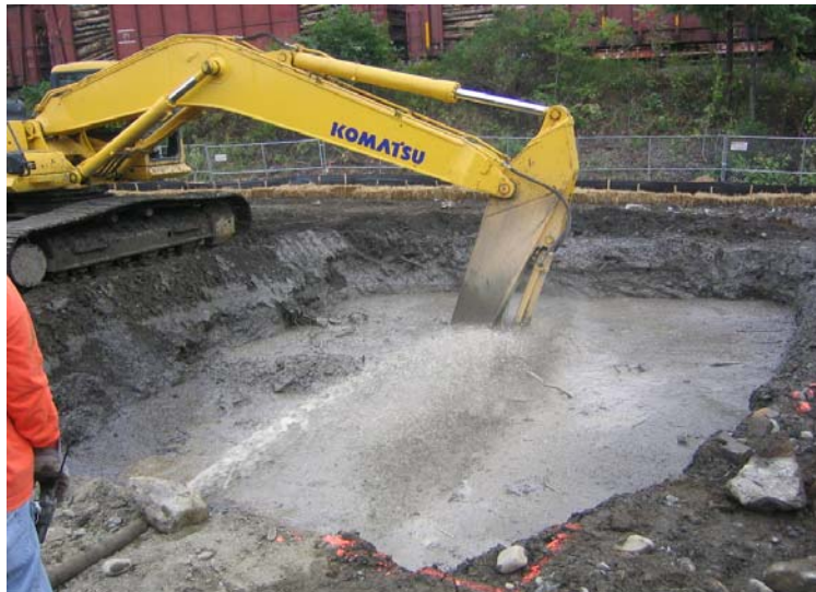
Figure 5. Excavator mixing
