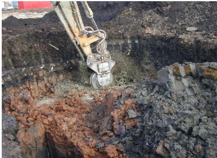
Figure 4. Rotary blender attachment
