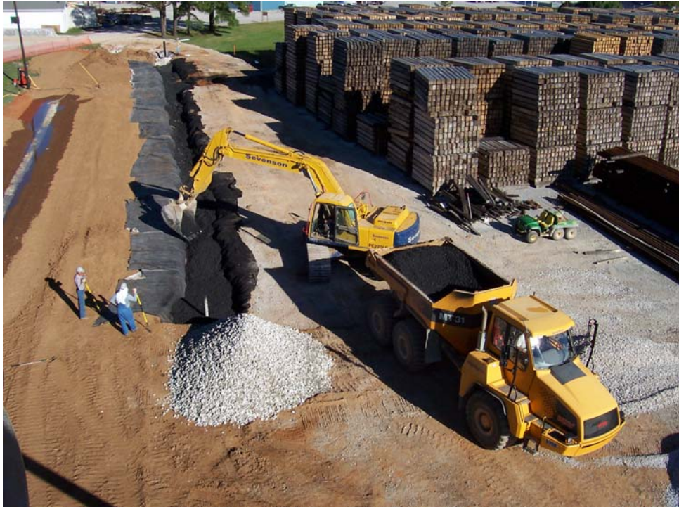
Figure 2. Passive DNAPL Barrier Trench Installation
