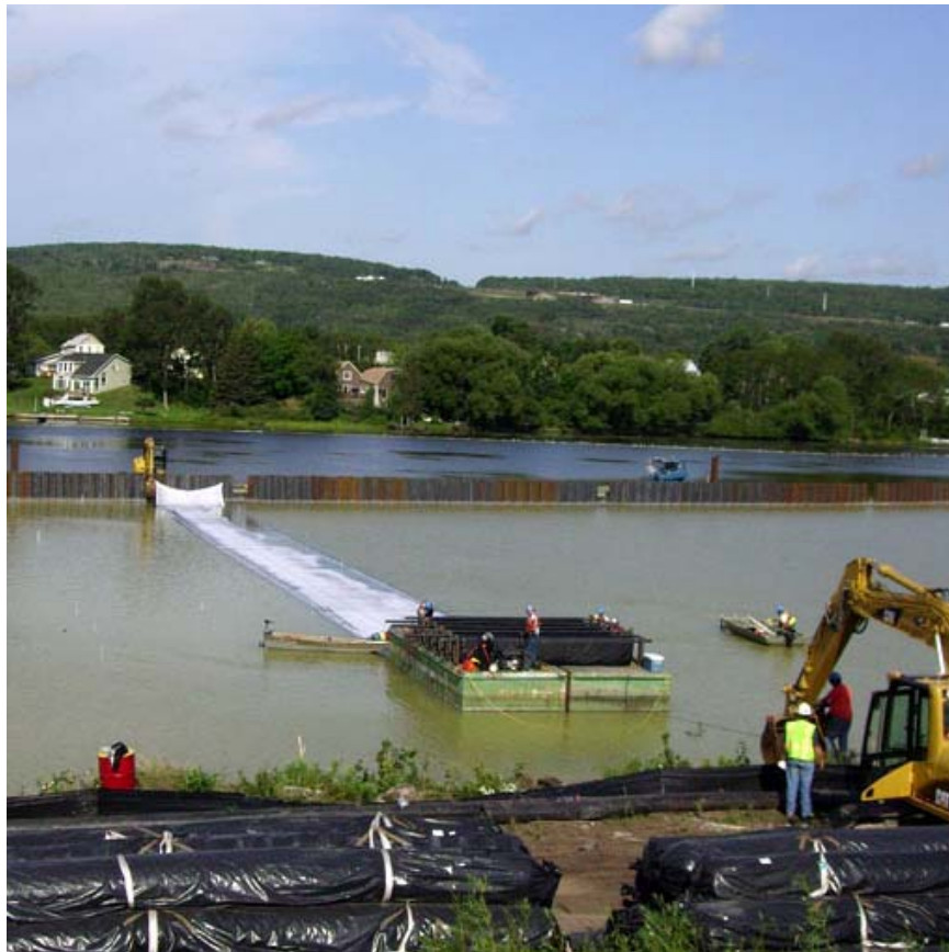
FIGURE 5. Reactive mat being deployed from barge.
