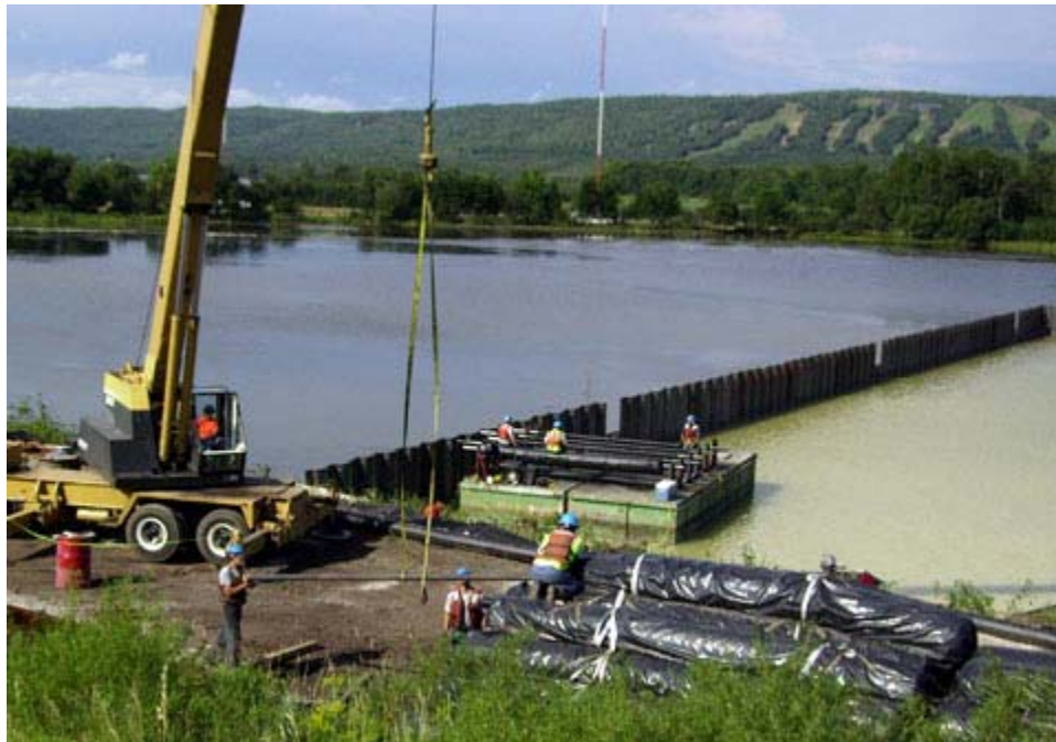
FIGURE 4. Reactive material mats being loaded onto barge.
