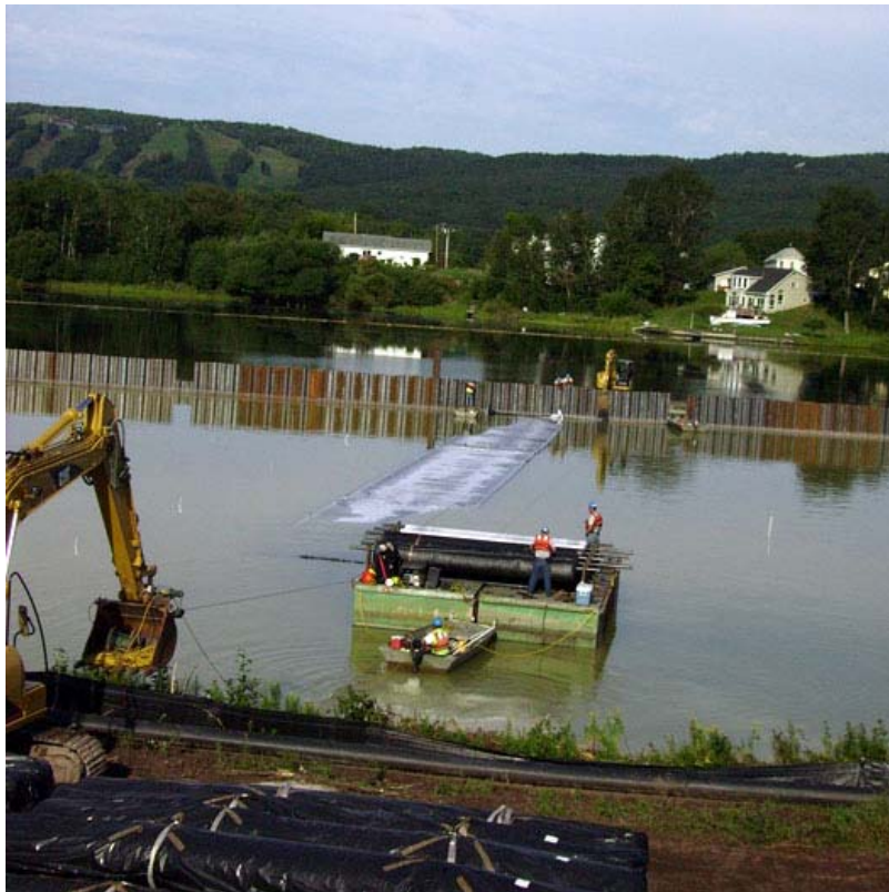
FIGURE 6. Barge being repositioned for next row of panels.
