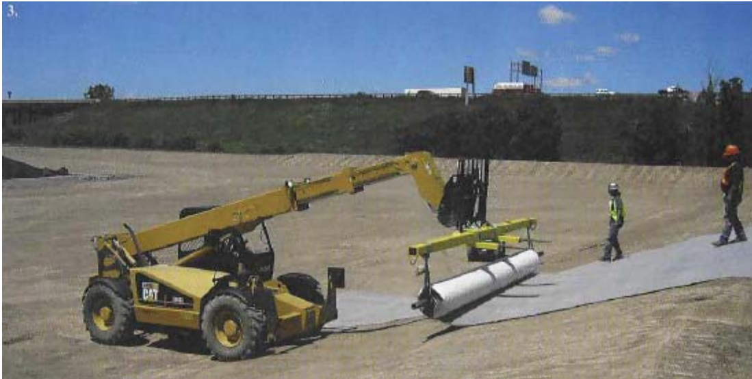
Figure 2. GCL being deployed over prepared subgrade.
