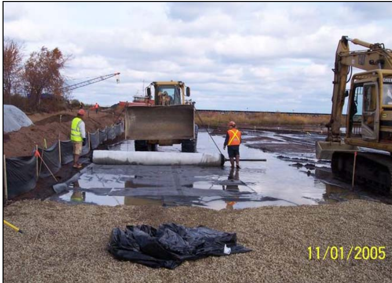
Figure 2. RCM deployment with front end load equipped with spreader bar system.
