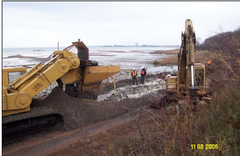
Figure 3. Continuous trenching of organoclay PRB.
