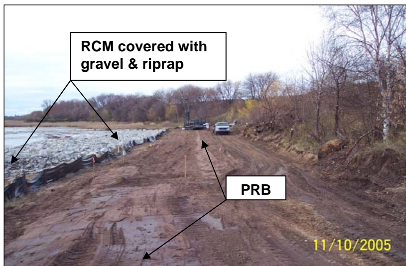
Figure 4. Alignment of organoclay RCM and PRB
