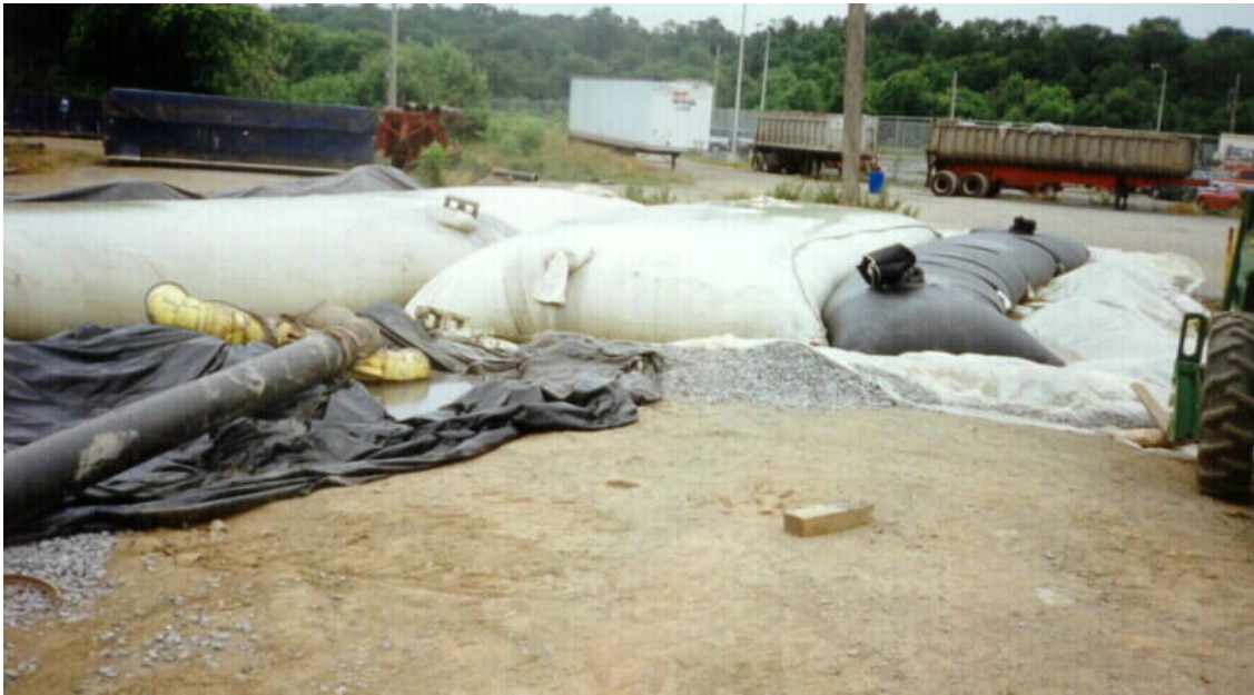
Figure 5 – On site dewatering of sludge within polyester and polypropylene geotextile tubes
