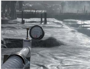
2. Starting Smoke Test
