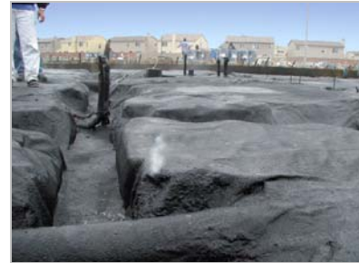
3. Puncture Detected
