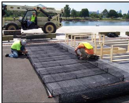
Mattress sections are filled with stone (stone size varies) and the geogrid is seamed shut. Reactive Core Mat is attached to the bottom of the mattress.
