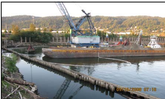
Placement of Organophilic Clay Nearshore Cap
