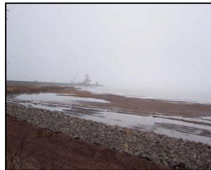
The finished PRB.
