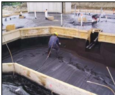
Liquid Boot® conforms to irregular surfaces and can be applied in the most challenging conditions.
