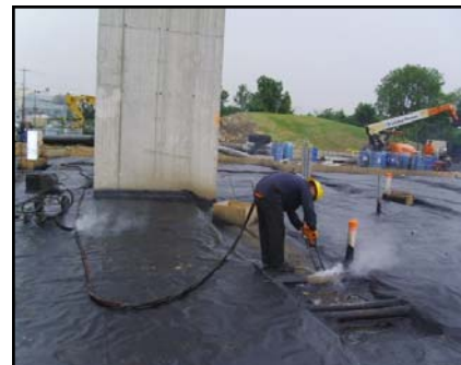
Liquid Boot® spray-application effectively and effortlessly seals around crucial areas such as pipe penetrations.
