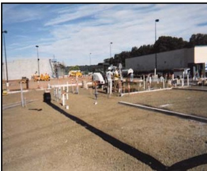
Liquid Boot® GeoVent trenchless gas venting system installation directly on the subgrade.
