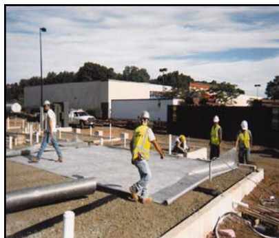
Liquid Boot® BaseFabric provides a uniform substrate for which the Liquid Boot® gas vapor membrane is then sprayed.
