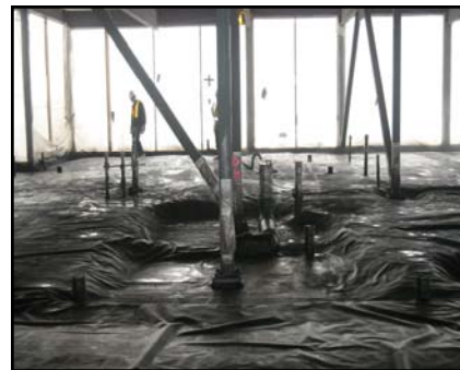
The installed spray-applied gas vapor membrane attaching to the piles themselves and conforming to the haunch.
