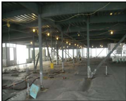
LIQUID BOOT® Base Fabric installation
