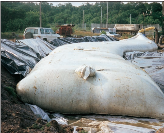
Tannery sludge is pumped from the holding tank into GEOTEX® Tubes.
